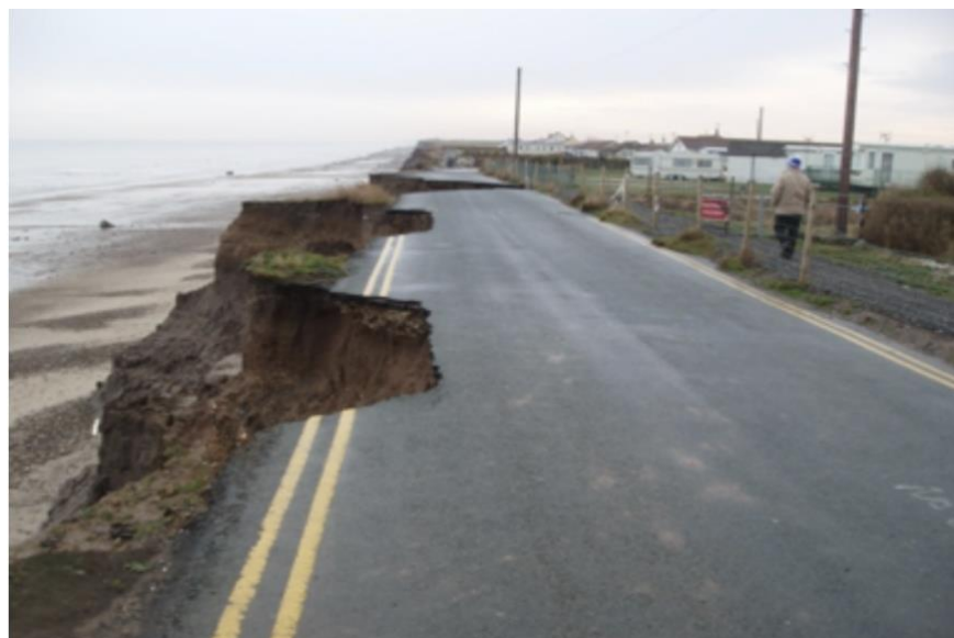
Figure 15 An example of coastal erosion showing the soft eroding cliffs at Ulrome in the East Riding of Yorkshire, UK. Photograph taken by Neil McLaughlin, East Riding of Yorkshire Council (12 May 2008). http://www.channelcoast.org/gallery/viewphoto/cliffs/soft_cliffs/1384
